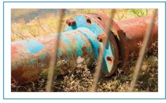
failures is the use of a coating with excellent barrier properties (to prevent the ingress of corroding species such as oxygen and water) and mechanical strength (to resist damage in the service environment).
